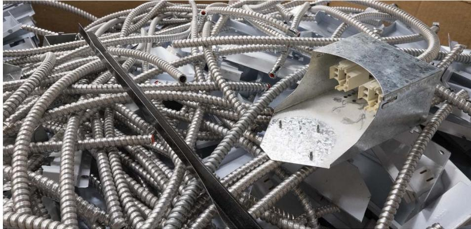
Removal of old lamp holders and ballasts at Terralux installation.
